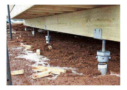
The City of Summerside accepts building permit applications for residential projects that include the proposed installation of helical piles (screw piles) that will be supplied and installed by companies whose products have a valid Evaluation Report by the Canadian Construction Materials Centre (CCMC). Since helical piles are not covered under the 2010 National Building Code of Canada, two documents are required to be submitted for all projects proposing the use of helical piles.
